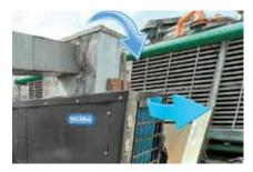
can be channel to cooling tower to improve its cooling capacity.
