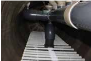
Internal plumbing & laterals
