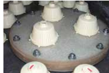
Internal Nozzle Plate Service Hatch
