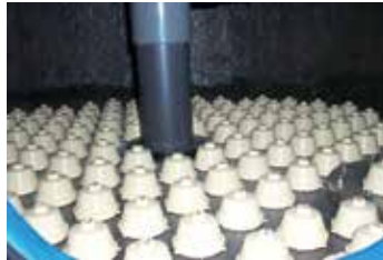
Nozzle Plate under drain system
