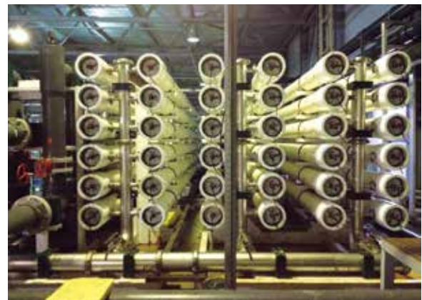
10,000 m 3 /d seawater reverse-osmosis (SWRO) desalination plant to support the drinking and process needs of local residents and the new Far Eastern Federal University.
