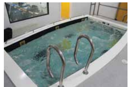
Wolves installed The SwimEx 600T paddle wheel resistance pool in 2005 for peak performance training and smooth laminar water flow for stabilised resistance physiotherapy.
