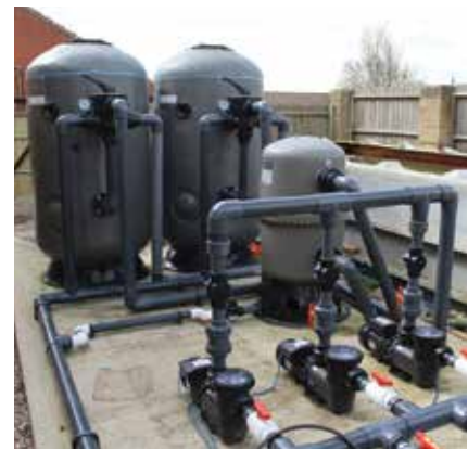
70XL Commercial MultiCyclone, two Micron SMDD 1050 fibreglass filters, three Hydrotuf pumps and glass media.
