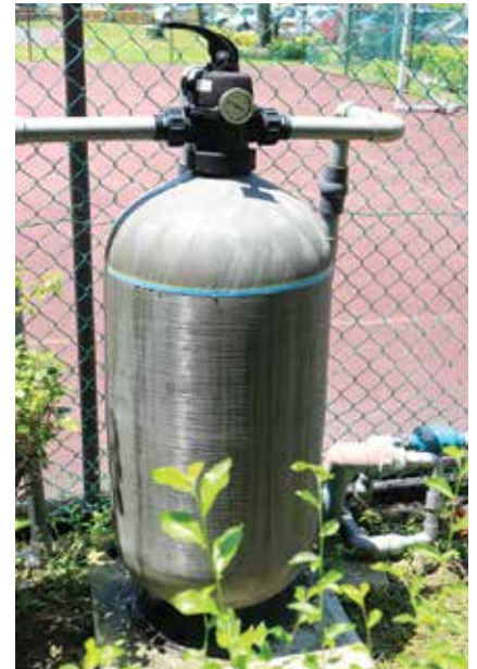
When you have children facing serious health challenges, clean, healthy water is essential to their recovery. A high quality filtration - Micron Deep Bed Sand Filter was recommended by Waterco as a solution.
