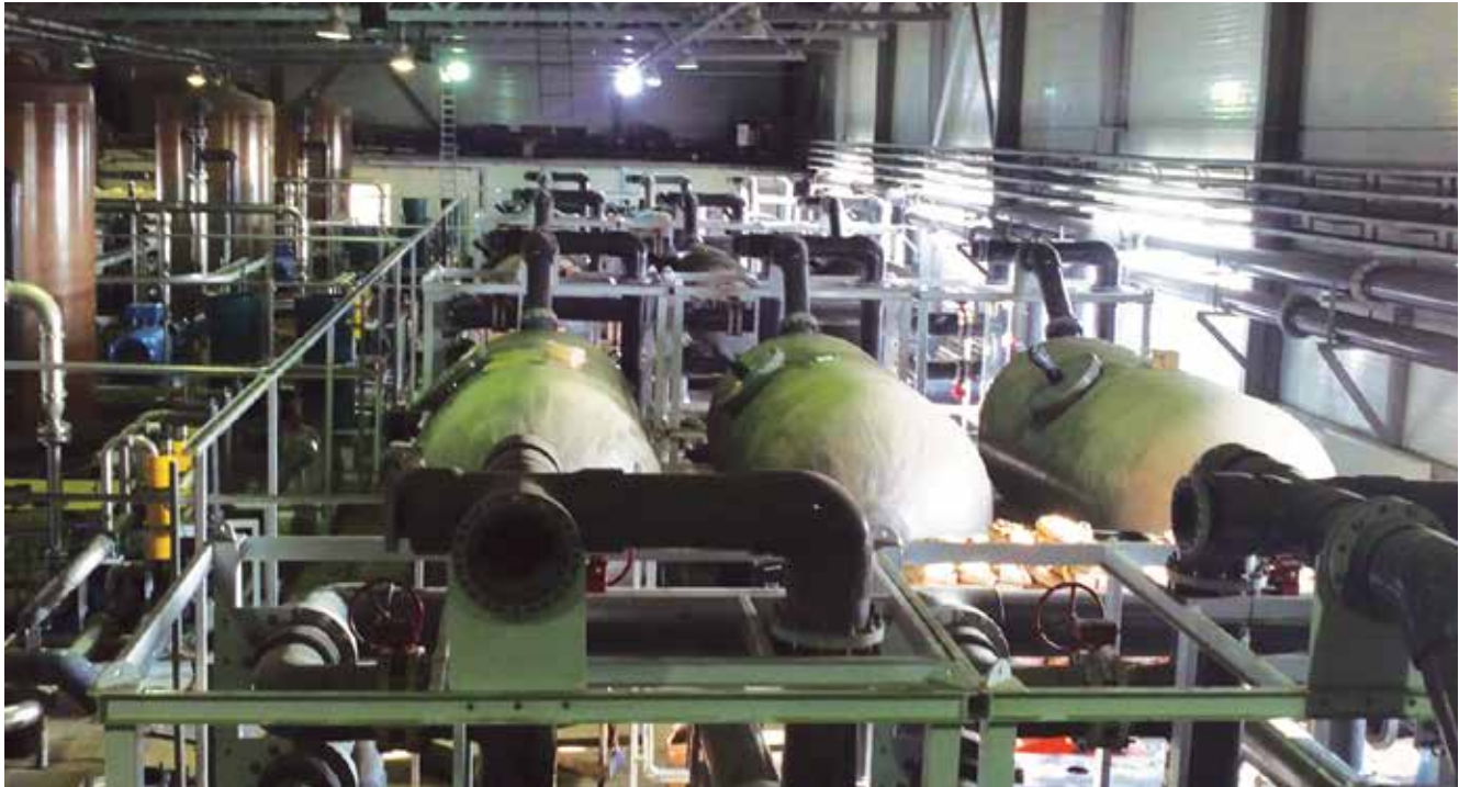
▲ Waterco was awarded the contract to provide 12 Micron MD10,000 horizontal filters. These 7-bar rated filters are made using the latest in fibreglass winding technology and use the highest grade of non-corrosive materials.
