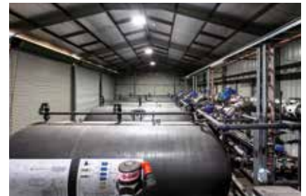
To deliver high-quality filtered drinking water free from unwanted taste and odours, Filtec installed Waterco's MPD10,000 Commercial Fibreglass Nozzle Plate Media Filter.
