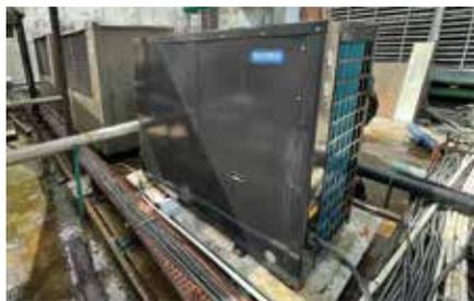
*Air to water heat pump with R417a refrigerant*
