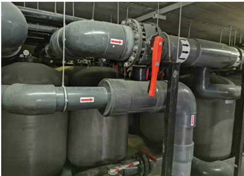
The original plant room consisted of four 2000mm horizontal filters
