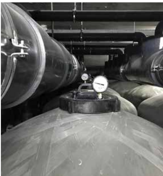
“Waterco SMD900h are easy to manoeuvre on to the site and install in the plantroom with minimal disruption to the hotel’s day-to-day operations.” Explains Jo
