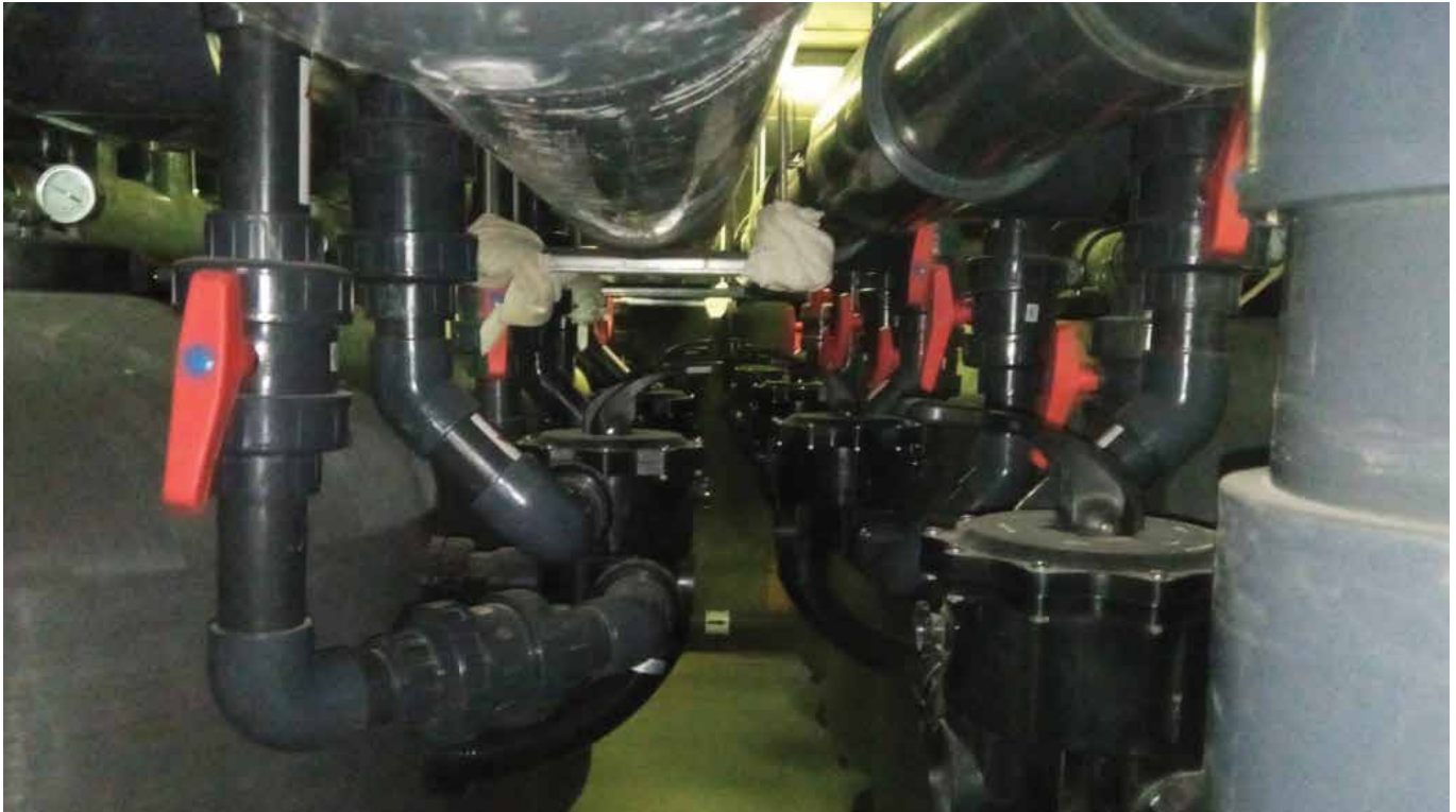
Compass – Those Pool Guys and Waterco were the only companies to offer a viable solution of fixing multiple small filters without disturbing the daily hotel activity in any way
