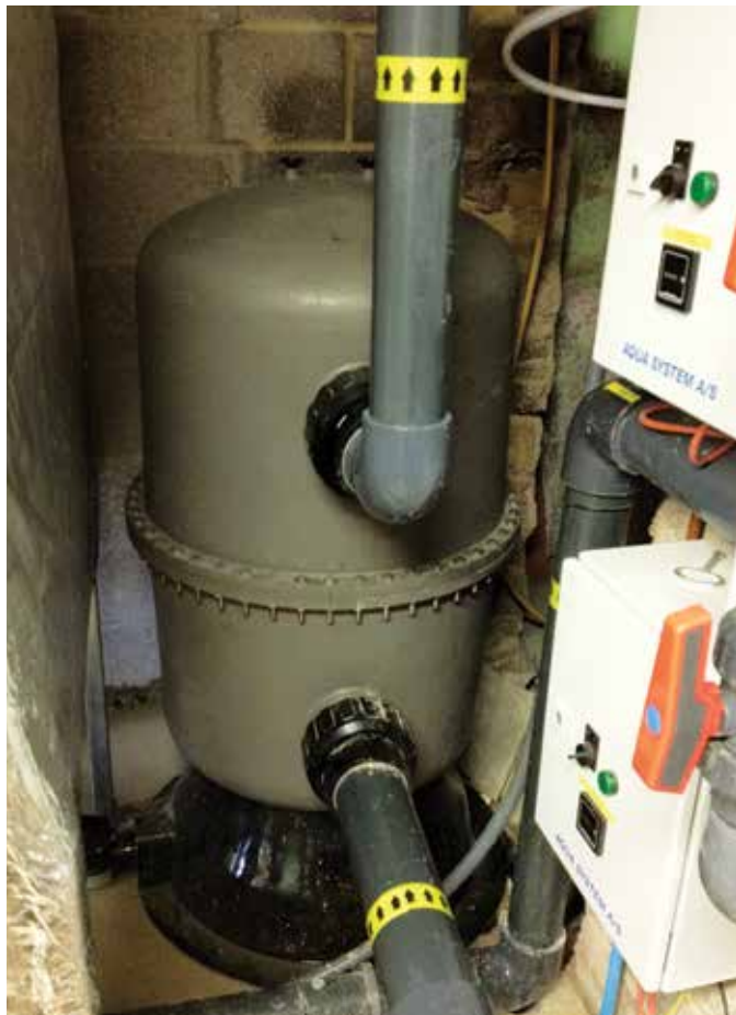
▲ MultiCyclone 70XL is capable of reducing filter maintenance and is ideal as a prefilter.
