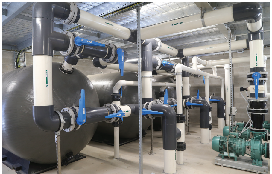
Waterco high-performance commercial filters were installed to provide consistently clean and hygienic water for students.
