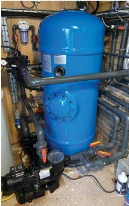
"Waterco's Lacron Deep Bed MBF filters were used due to the confined area of the plantroom" Bishop explains.
