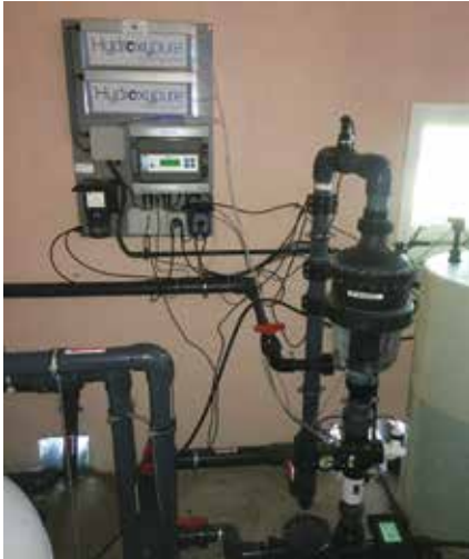
Hydroxypure sanitisation is based on the Advance Oxidation Process. (AOP), which combines Perox, a chlorine free sanitiser (H 2 O 2 ) and hybrid ozone (O 3 ) to create one of the most powerful oxidisers in nature.
